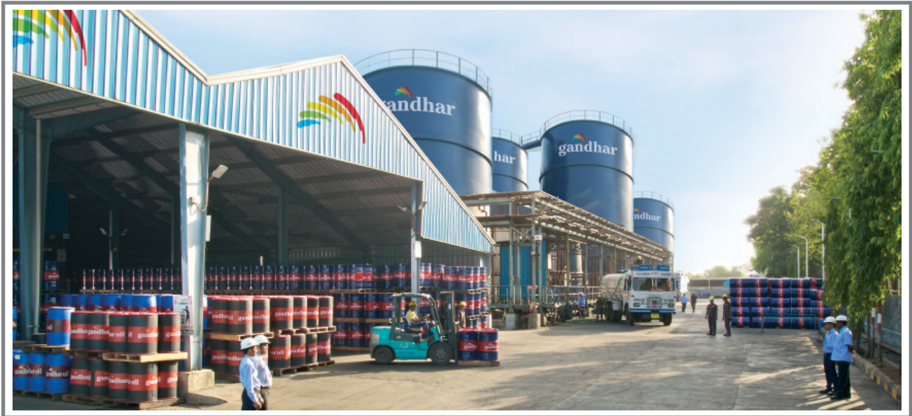
Storage tanks and drums at warehousing facility
